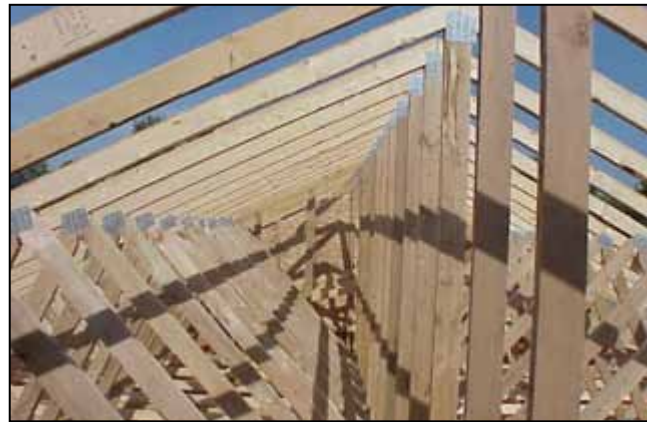
Figure 3.33. ~ Roof trusses containing hardwood lumber web stock.
