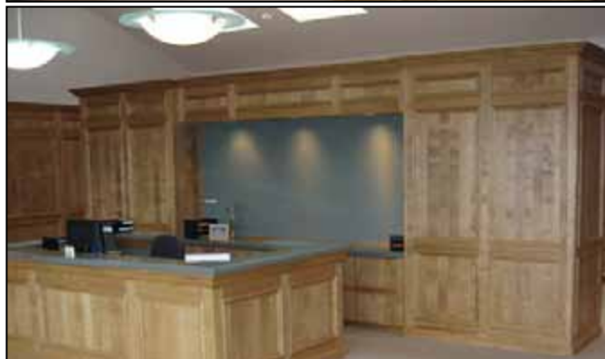
Figure 3.11. ~ Black ash engineered plywood panels and solid wood were used in this office. Photos courtesy of Scott Wothe.
