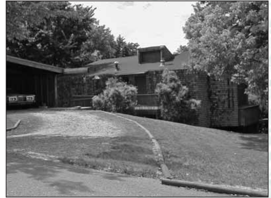
A wildland/urban interface with vegetation too close to wood siding.
